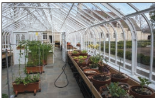
The original splendor of the greenhouse has been lovingly restored. The gardener's cottage, now repurposed as a guest house, is visible beyond.
