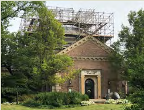
Lake Forest Library Dome Restoration
